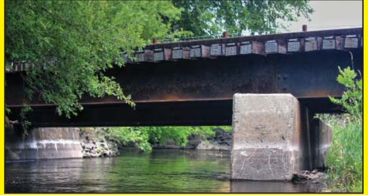
The Rail Road Bridge near the Toy House
